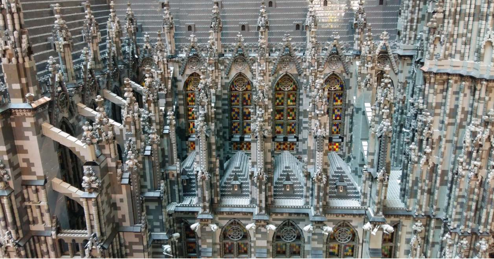
A look at one of the sides of the building, showing the windows and flying buttresses lining the walls.
