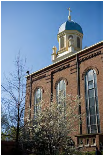
A side view of the church, showing the bell tower and windows.
